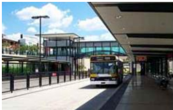
Figure 4.5: Brisbane South Eastern Busway
