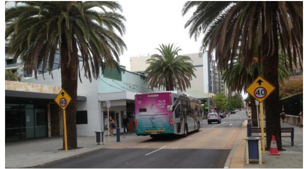
Figure 6.11: Raised platforms, Hay Street, Perth
