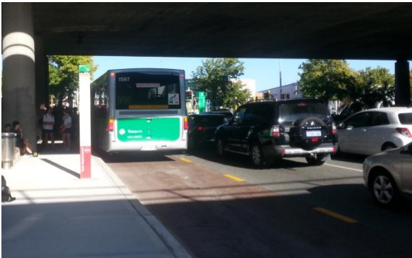
Figure 6.6: Bus embayment at timed stop outside Glendalough Train Station
