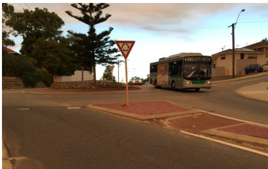
Figure 6.13: Typical Roundabout on bus route, Pearl Parade, Scarborough
