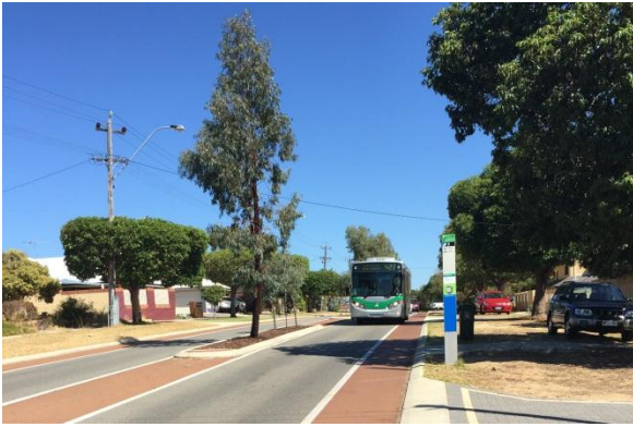
Figure 6.5: Bus stop on carriageway, Barnes Road, Innaloo
