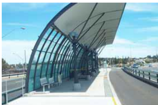
Figure 8.1: Bus Shelter at Canning Bridge Station
