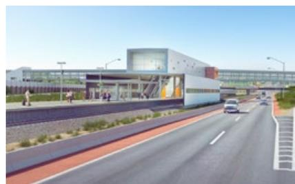
The station features the orange colour used to depict the Mandurah Line. The modular design is particularly important, as the station is being built in the middle of an operating rail line, and the Kwinana Freeway.
