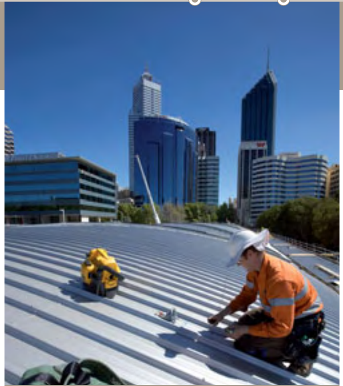
Roof construction at Esplanade Station, part of the new Southern Suburbs Railway.
