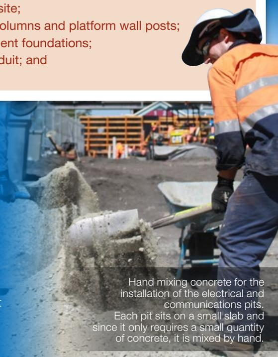
Hand mixing concrete for the installation of the electrical and communications pits. Each pit sits on a small slab and since it only requires a small quantity of concrete, it is mixed by hand.
